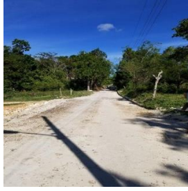
Section of rehabilitated road, Queenshythe (St. Ann)
