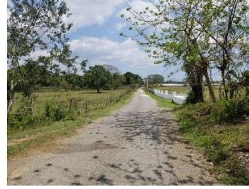
Section of rehabilitated road, Spring Park (St. Elizabeth)
