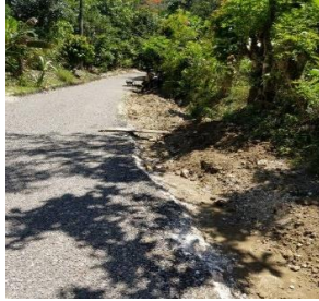
Section of rehabilitated road, Cocoa Walk (St. Catherine)
